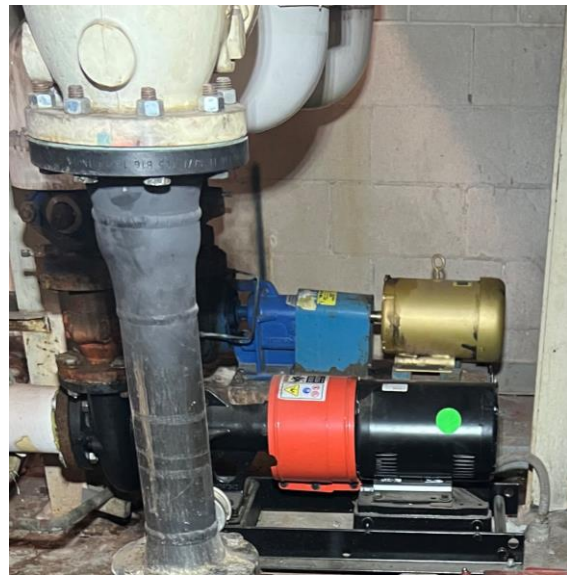
Picture 8: Chiller #2 Condenser Water Pump (P-7)
