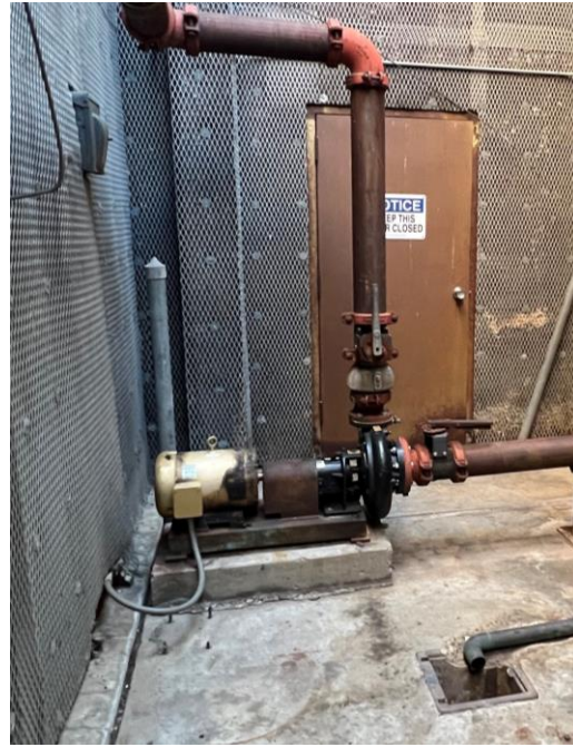
Picture 8: Chiller #2 Condenser Water Pump (P-7)
