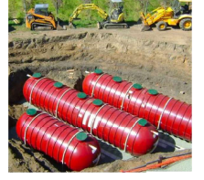
PROPOSED 30,000 GAL XERCES UNDERGROUND TANK - 10' X 54'
