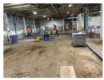
Preparing for new concrete slab after seismic stabilization.
